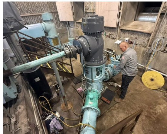
Installing Rebuilt RA Drive at PP1-E2
