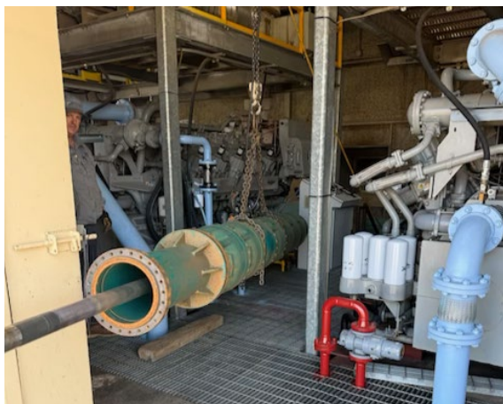
7 Stage Pump Removal at PP1
